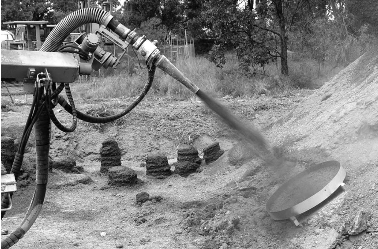
FIG. X1.6 Remotely-Controlled Spraying of Panels
