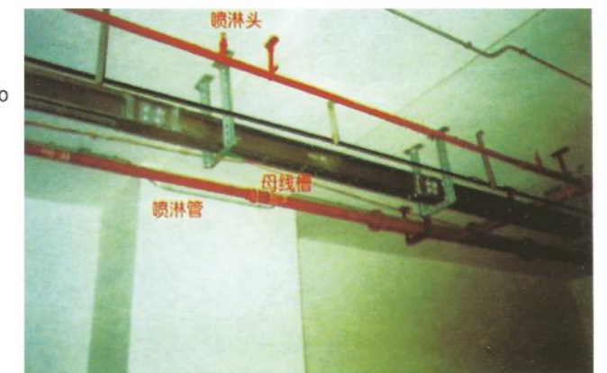
防喷水防水母线槽在工程中应用实例 Defend spraying water and apply the embodiment in project with waterproof bus bar trough
