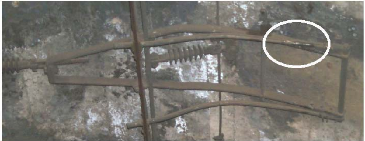
Figure 2: Cause of vertical impact force due to pantograph hitting cross-span. This was due to low tensioned OHTE causing abnormally high contact wire uplift.
