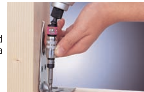
Installing tension and angle brackets
