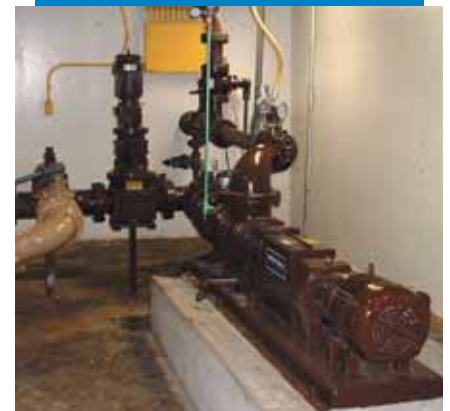
A Moyno Pipeliner grinder and a 2000 pump are teamed in this primary sludge transfer application. Moyno has the breadth of product offering needed to provide effective, packaged application solutions.
