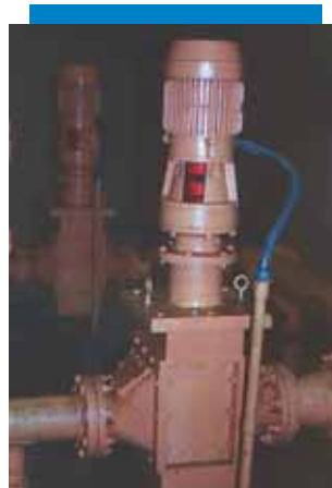
The Moyno Annihilator utilizes advanced, proprietary cutting technology in shredding solid objects and materials that are often suspended in raw wastewater to reduce them to a more manageable size. They are available in flanged and open channel configurations.
