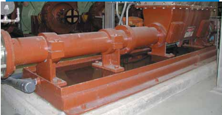
This Moyno 2000 G2 scum transfer pumping system was specifically designed for one of the largest wastewater treatment plants in the midwest United States. Moyno engineers worked closely with city engineers to design and manufacture 18 systems to satisfy specific, critical application requirements.
