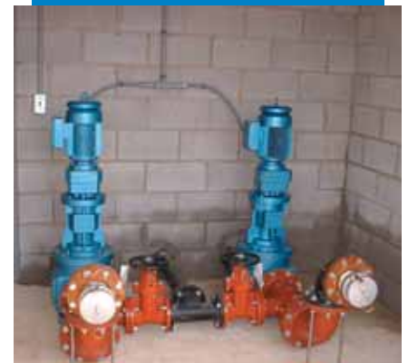
Moyno Pipeliner single shaft grinders reduce solids to a consistent, manageable size to prevent clogging, ragging and damage to downstream equipment.
