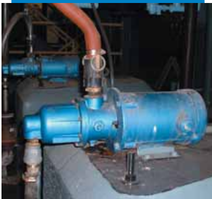
The low shear pumping characteristics of the Moyno pump make it ideal for polymer metering applications.
