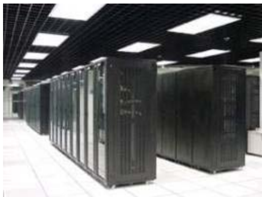
IDC机房 --- KYXBXZ-B & KYXBQ-200/400V-4L
