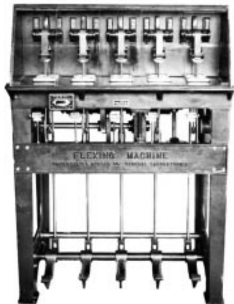
FIG. 1 Scott Flexing Machine with Five Hubs
