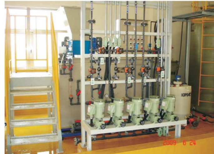
PAM自动溶解投加装置 PAM automatically dissolved dosing device
